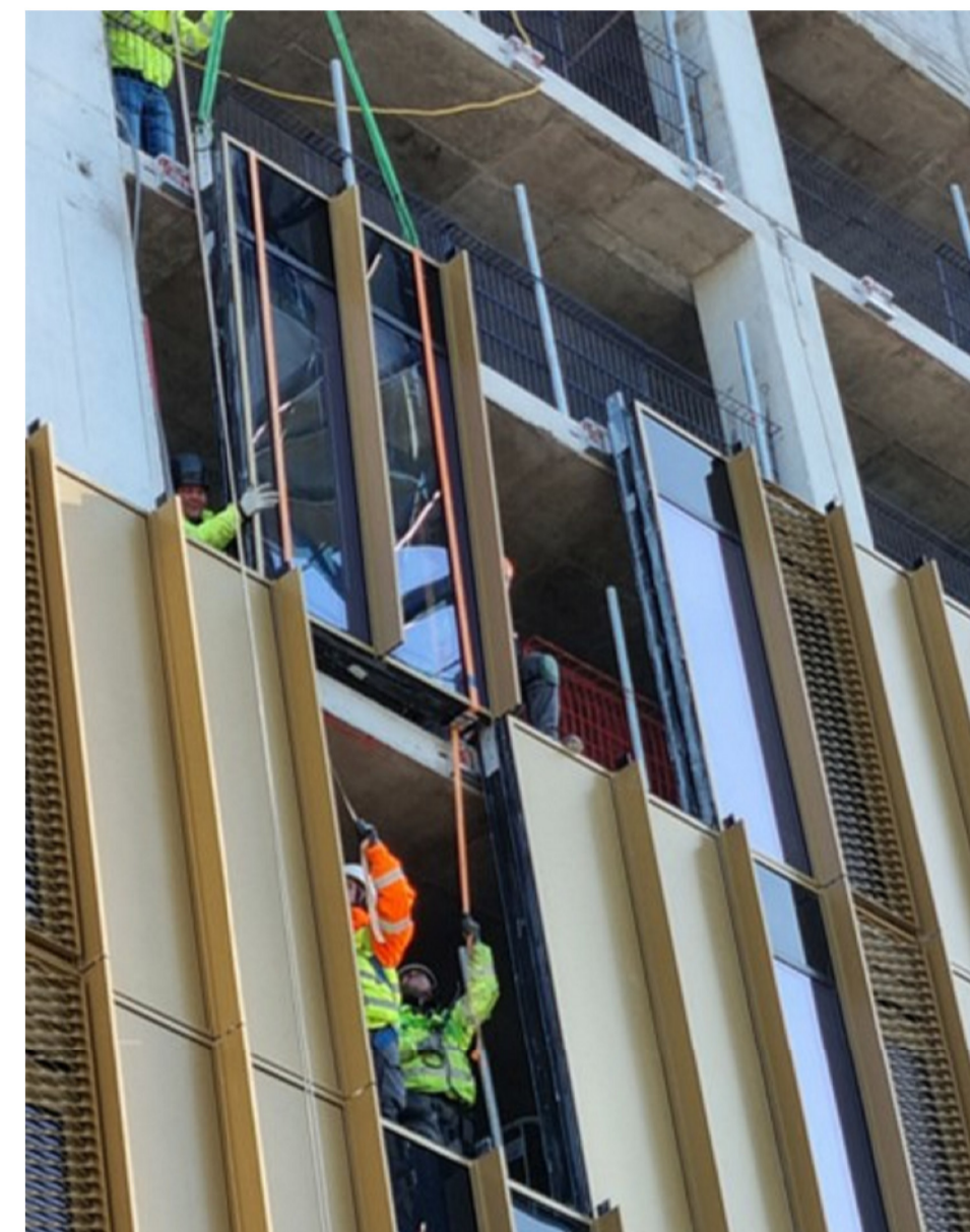
UNITISED CURTAIN WALLING UNDER CONSTRUCTION
