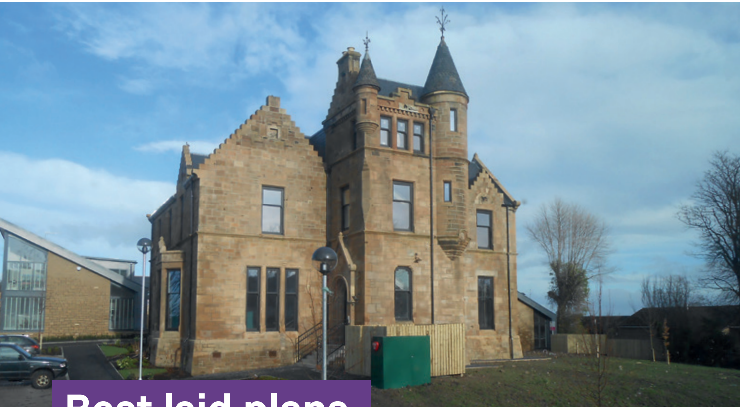
The completed project
