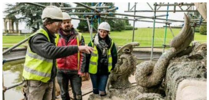
Figure 9: Assessing the conservation, repair and maintenance (CRM) requirements for Witley Court Fountain
