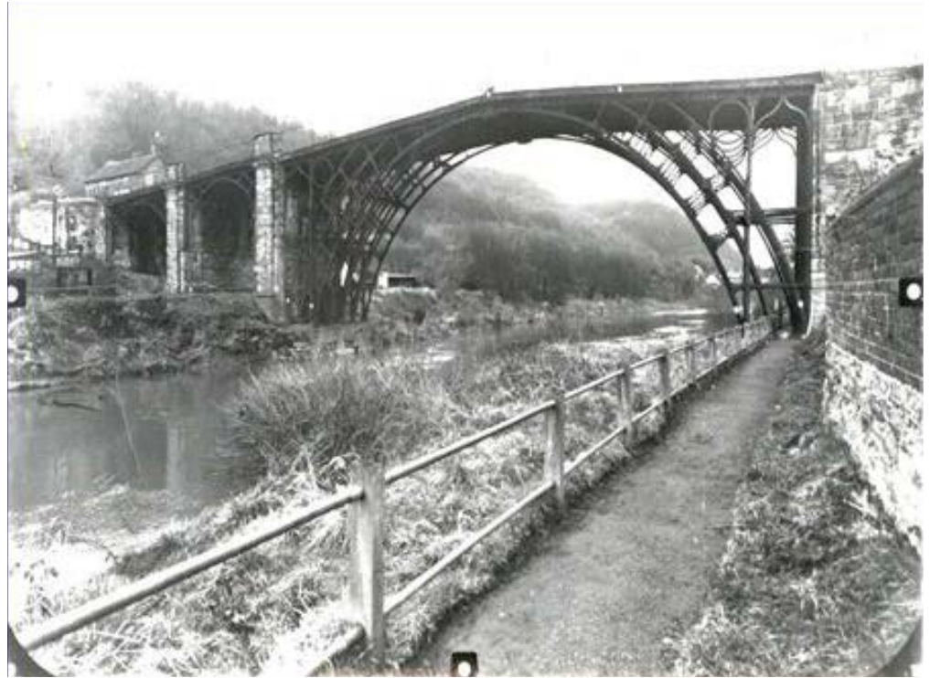
Figure 16: Archive photograph of the Ironbridge captured during photogrammetric survey work from 1972
