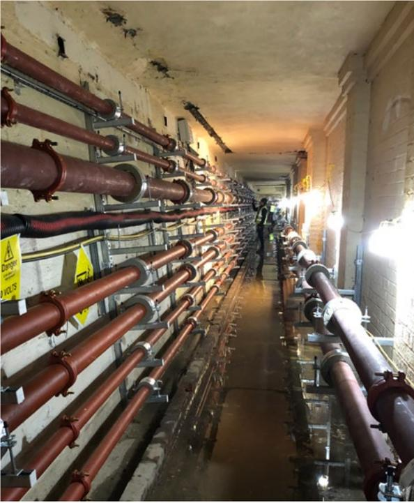
secured by a coupling which houses a resilient, pressure-responsive elastomer gasket. The coupling housing fully encloses the gasket, reinforcing the seal and securing it in position as the coupling engages into the pipe groove. Only two nuts and bolts are needed to secure the self-restraining joint. The mechanical joint creates a triple seal due to the design relationship between groove, gasket and housings, which is enhanced when the system is pressurised.
