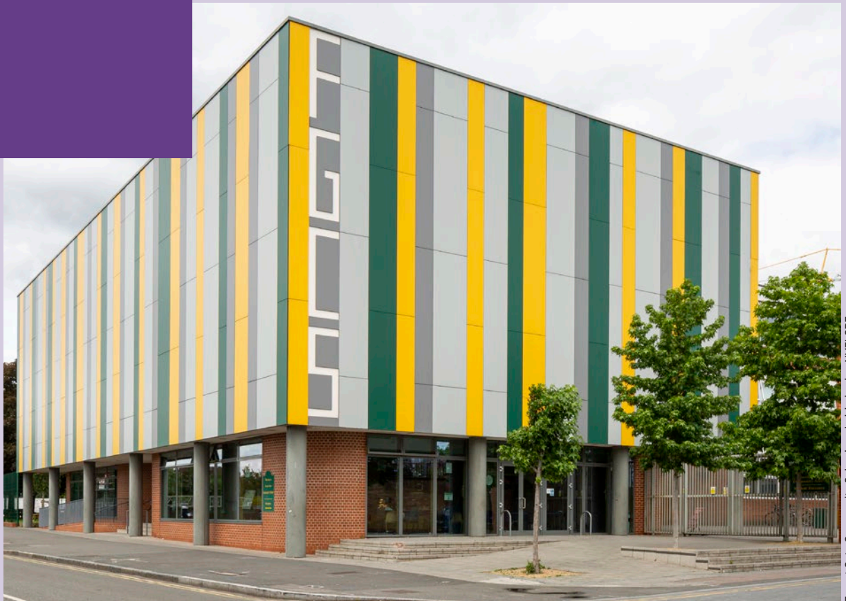
Forest Gate Community School, recladded using NVELOPE products and brackets.
