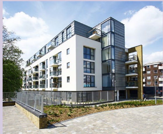
Packington Housing Estate in Islington transformed through NVELOPE's building envelope solutions
