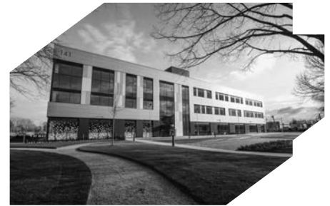
141-143 Park Drive East, Milton Park SRA Architects
