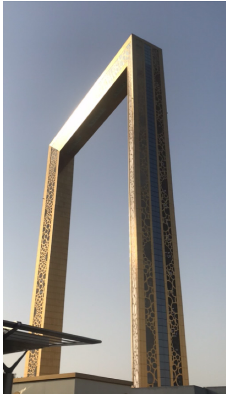
The Dubai Frame: Designed by Fernando Donis, 2013
