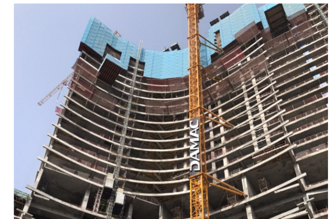
Damac Tower under construction
