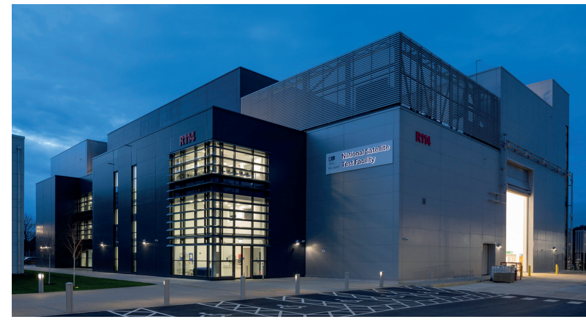
▲ NSTF Building Exterior
