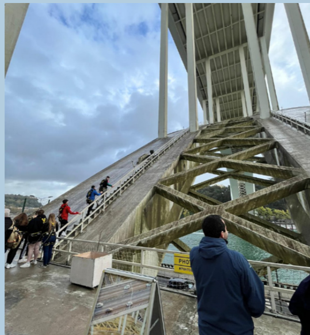
Arrabida Bridge arch
