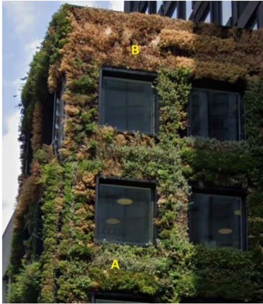
One example of a UK living wall installation with obvious variations in condition. The part marked at “B” is likely to fall well outside the condition of the lab tested samples and likely to surpass the minimum surface spread of flame requirement of ADB as it could be a class D or even an E!
