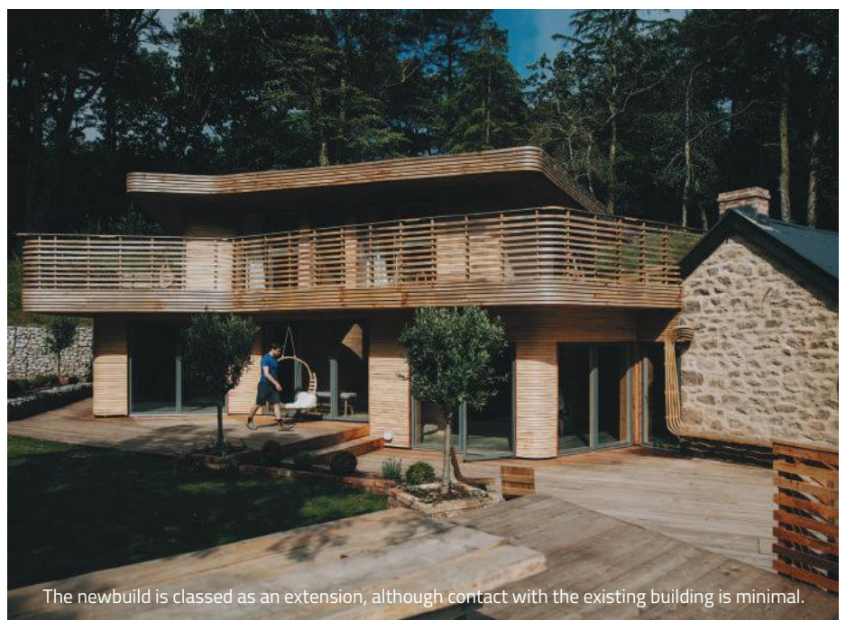
The original Georgian cottage was cleverly linked to the new structure (below and opposite) to gain planning approval.
