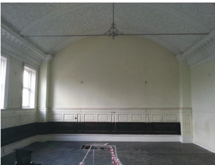
Lecture theatre before refurbishment
