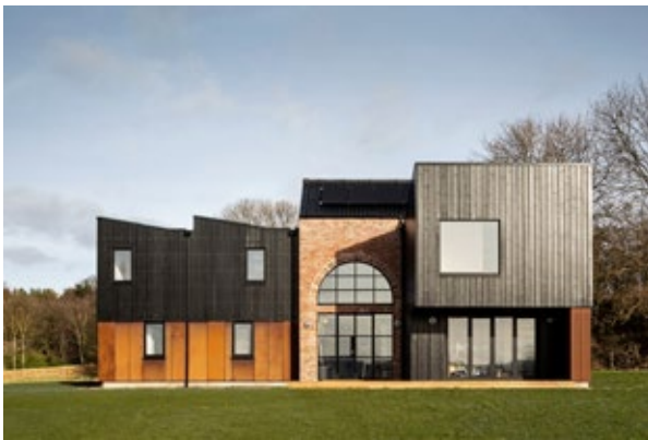
Fife Architects designed Iron Mill Bay House to perform as efficiently as possible in terms of energy and impact on the environment. The team created a highly insulated house using renewable energy sources including an air source heat pump and a rainwater harvesting system. © Keith Hunter
