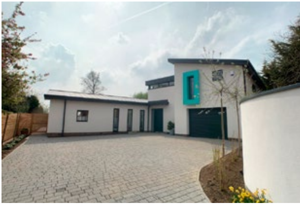
Designed by BRP, the central atrium at APRA House has high electric windows to draw out warm air during the summer months. Meanwhile, the roof extends over the southerly glazing to offer shading from summer sun, whilst allowing the lower winter sun to enter deeply into the space benefitting from the solar gain.
