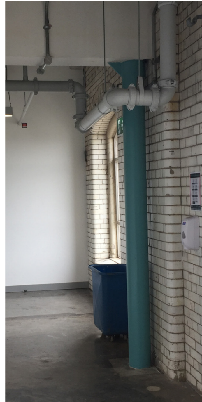
CHS column fed between floor plates
