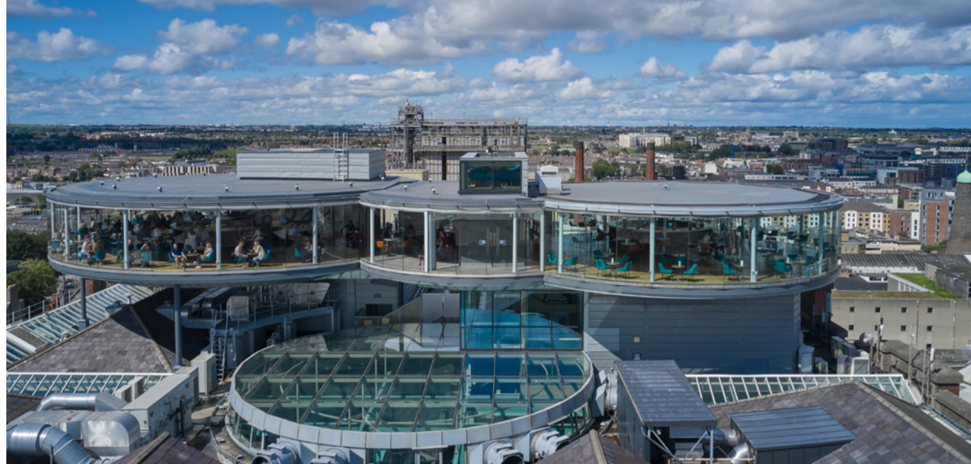
Aerial photograph of Gravity Bar Expansion overlooking Dublin City
