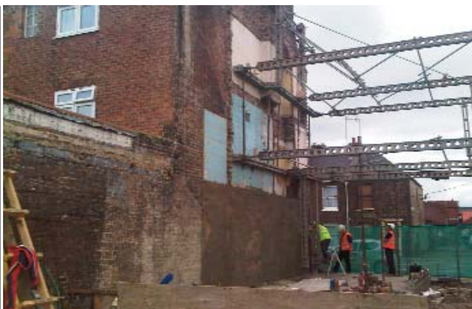
This page and opposite: Mabeys support system used to support dwellings either side following demolition of an attached terraced property. Party Wall Awards were put in place and a
