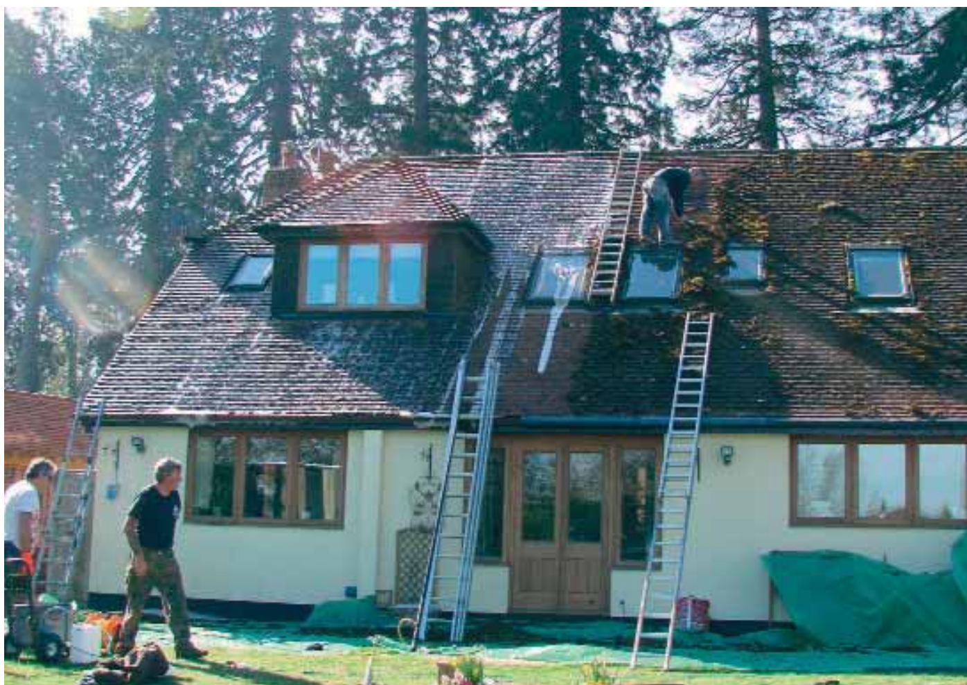
Above: specialist cleaning of heavy mould formation on clay tiles.
