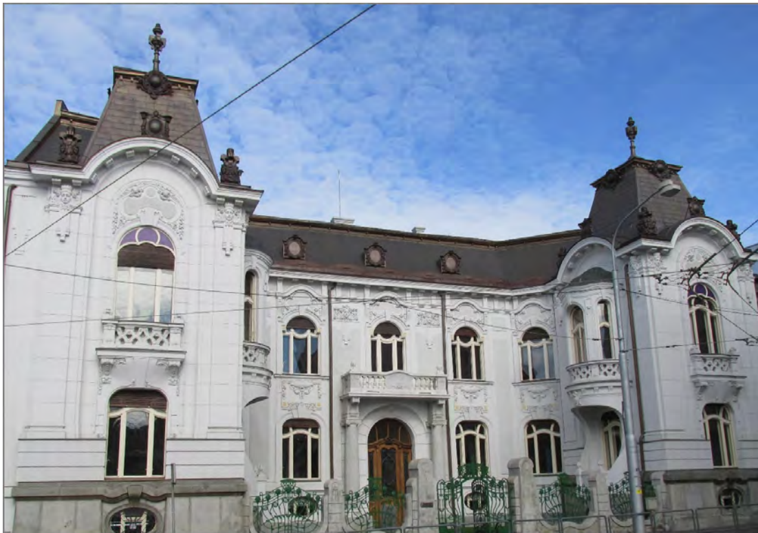
Rosenfeld's Palace Restored in 2016 with new Copper Roof
