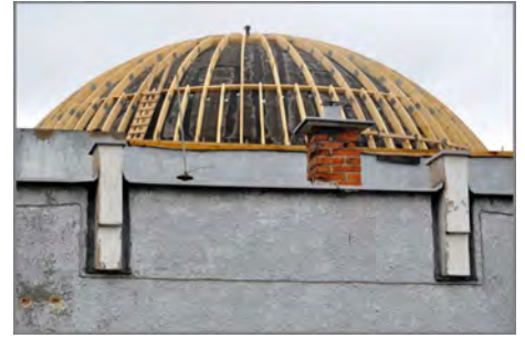
Primary dome rib framing.
