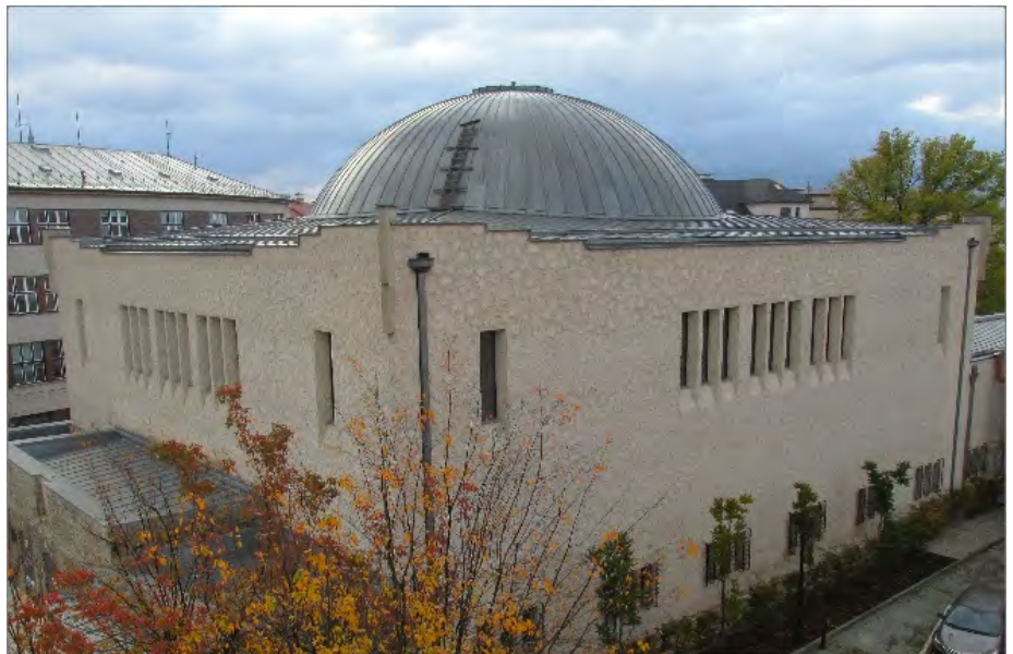
The New Synagogue with completed dome.
