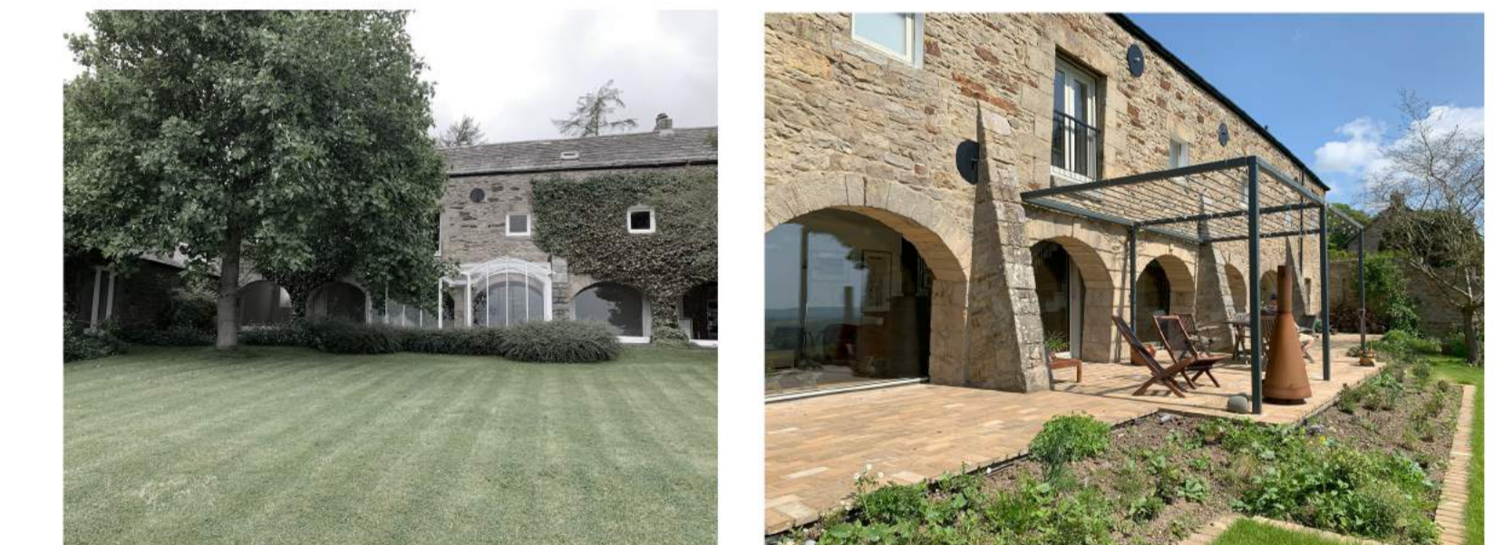
Existing - South Garden
