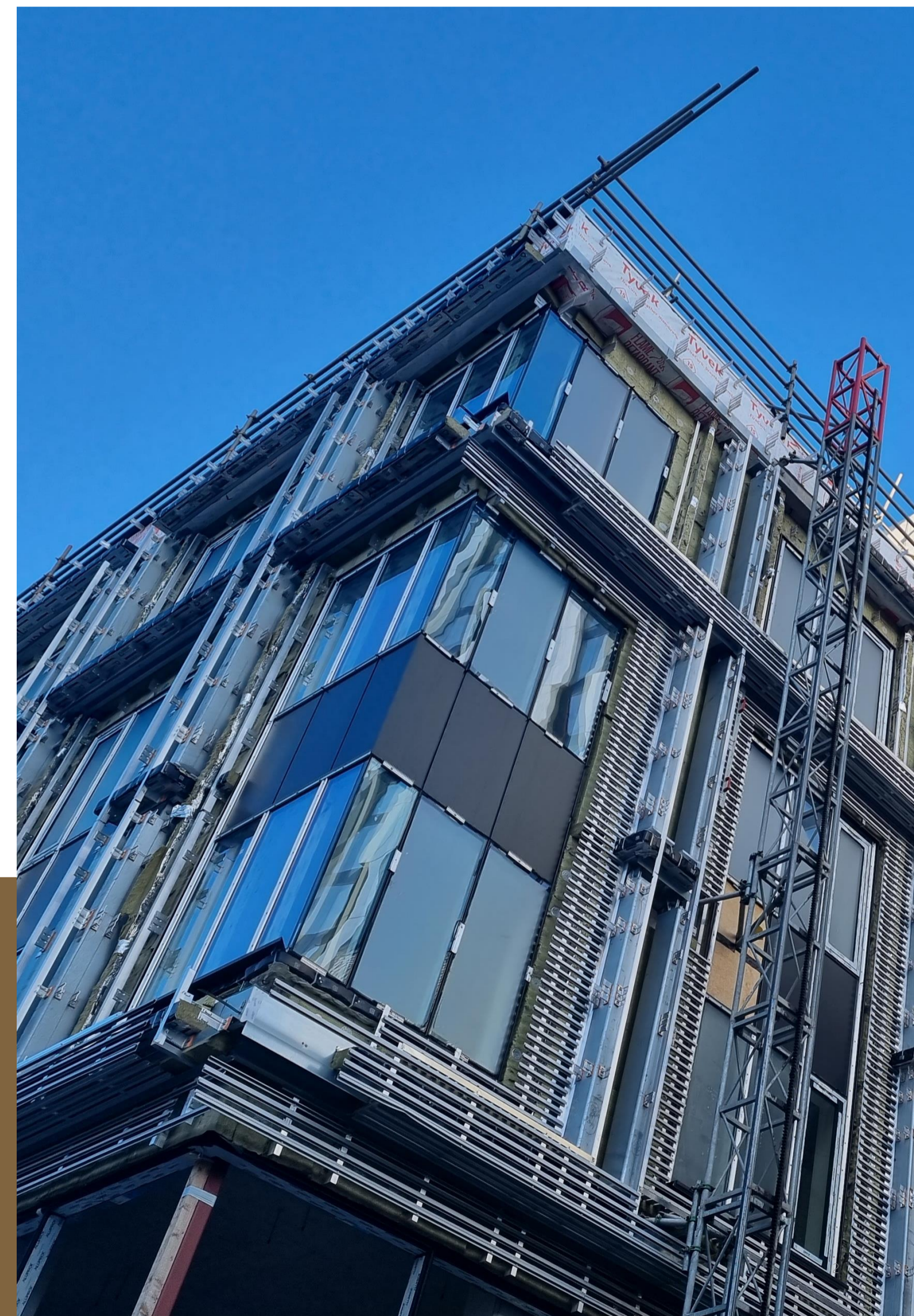
Brick slip cladding being installed to for deep reveal façade.
