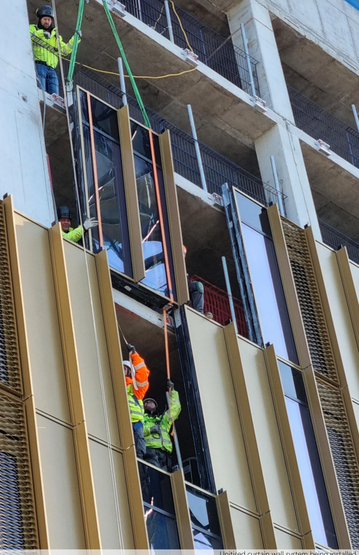
Unitised curtain wall system being installed
