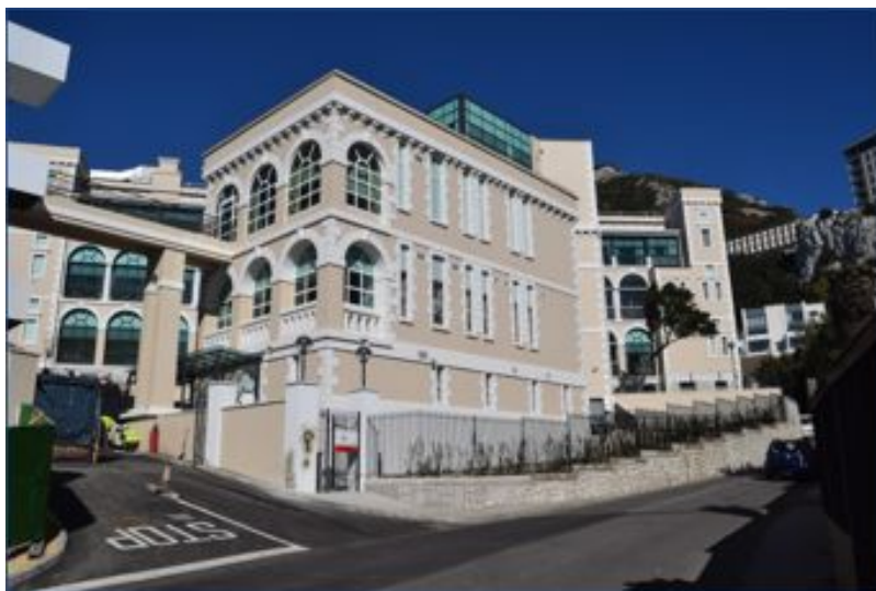
Royal Navy Hospital. Refurbished into elderly care and mental health facilities.
