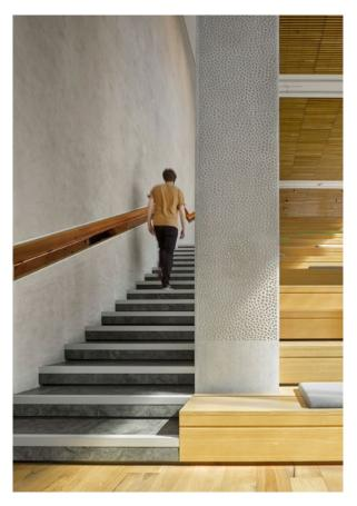
at 1:1 scale to understand what the pattern would look like and Reckli then gave input into the depth and shape of the holes which would be suitable for striking the shuttering from the concrete. Once the Grasshopper model had been updated to reflect this, 3D models were supplied to Reckli
