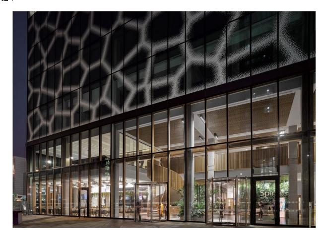
such as the curtain wall façade system – the Voronoi pattern, but also internal timber cladding along mullions and transoms, to continue visible connectivity to nature. Other references are exposed concrete columns which are moulded to reflect the trabecular system within human bones, which is the strongest part of a bone for reflecting mechanical stress.
