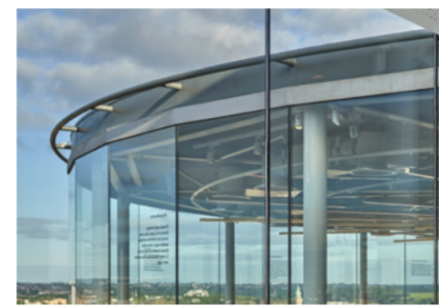
photograph of glazing roof interface
