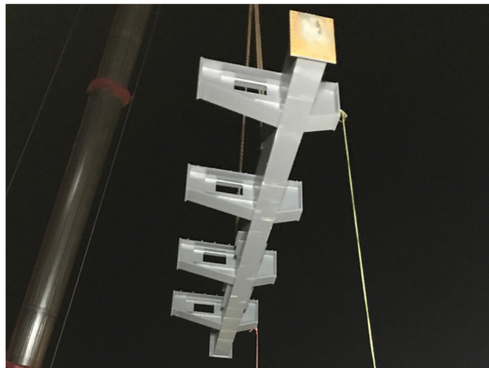
photograph of night time lift of girder structure
