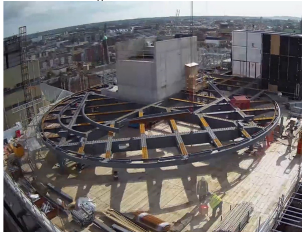
aerial photograph of steel structure during construction
