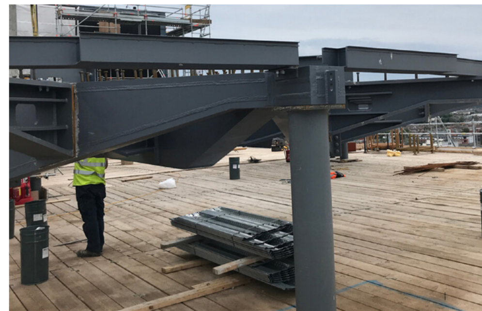
photograph of steel structure during construction
