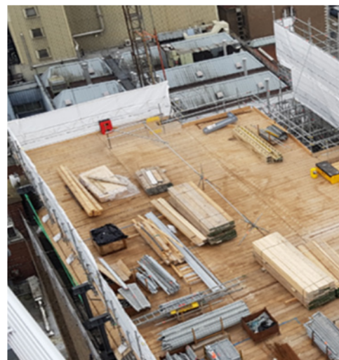
photographs of crash deck during construction
