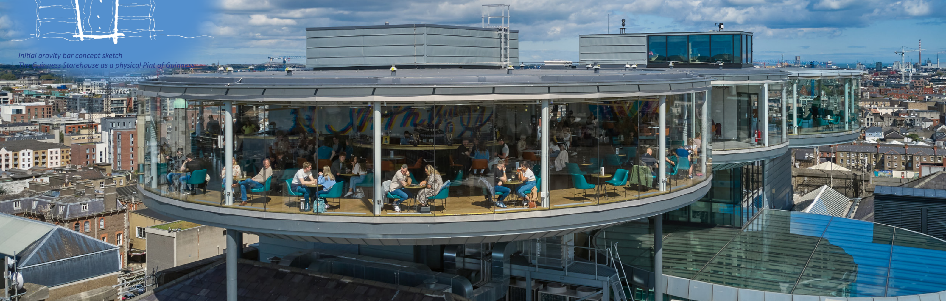
aerial view of finished extension
