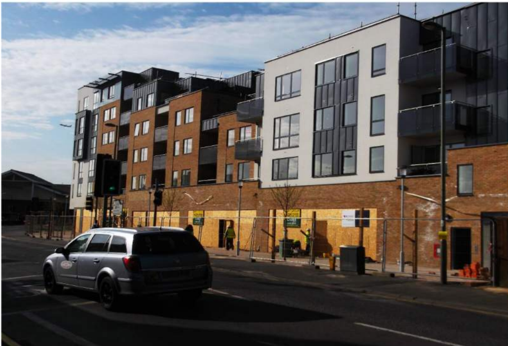
Newman House, finished project
