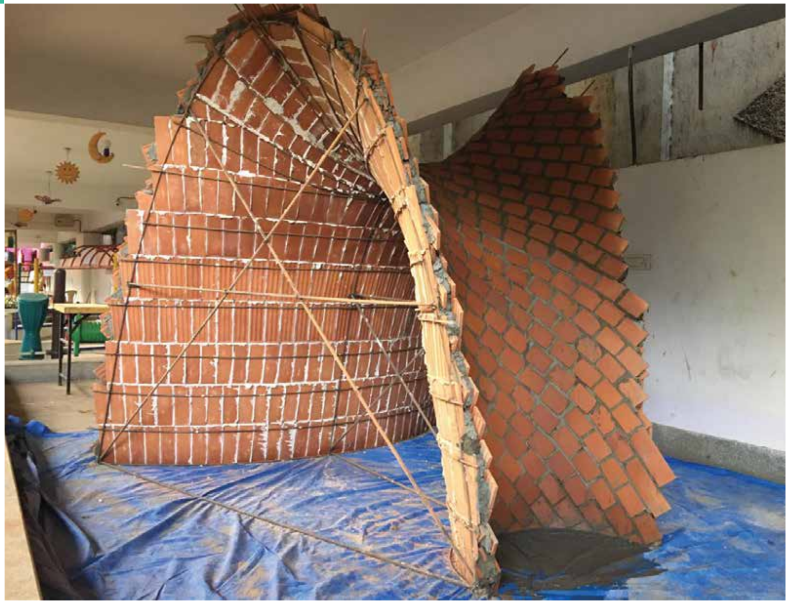
Brick vault made at site by Ar. Senthil Kumar.
