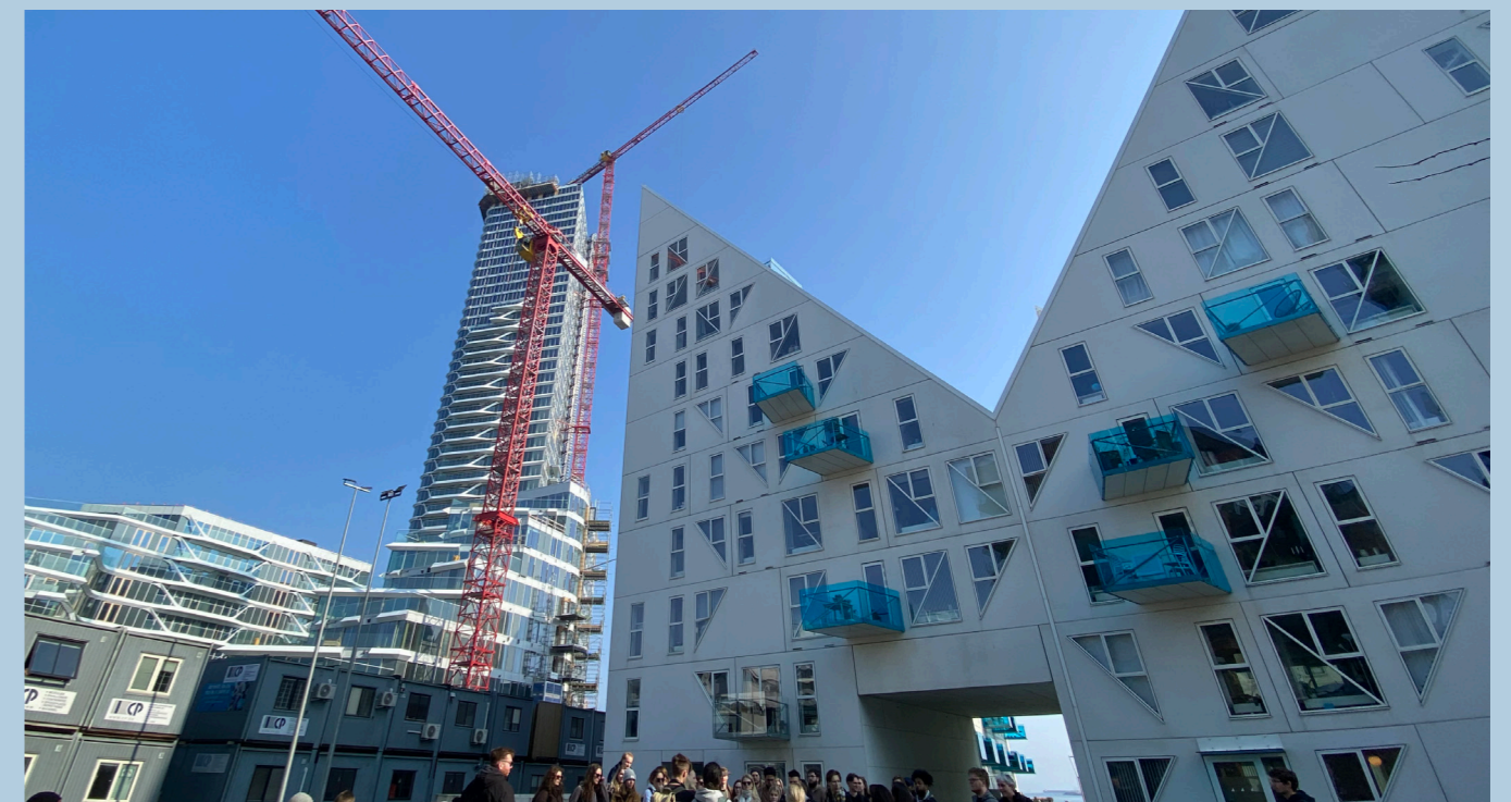
The Lighthouse construction with The Iceberg development in the foreground
