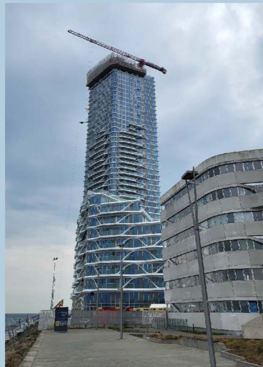
The Lighthouse currently under construction
