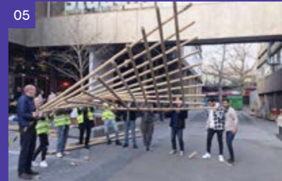
05 Testing the weight of the tensegrity bamboo roof!
