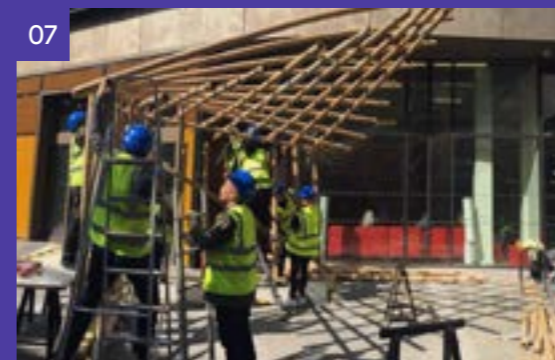
07 Securing the bamboo tensegrity roof onto the structure and foundation.
