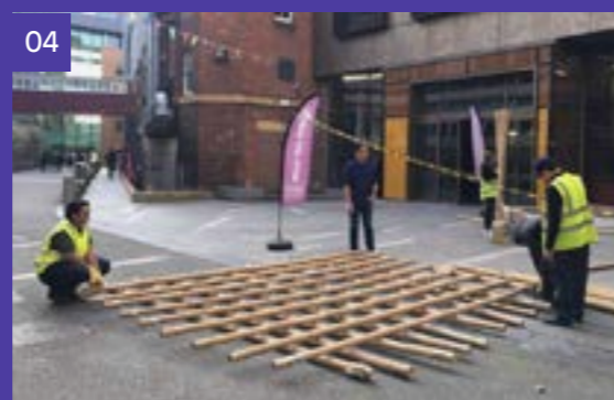
04 Putting the tension on the tensegrity structure.
