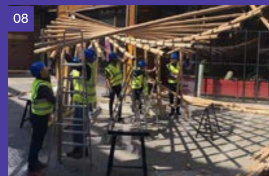
08 The roof is up and floating!
