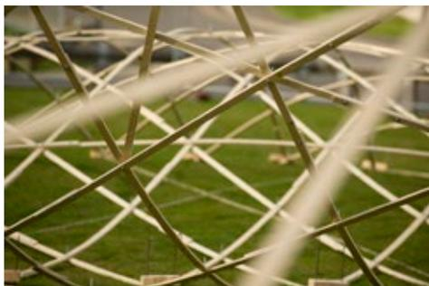
In 2016, to mark the Festival of Making in Sheffield, UK, a lightweight gridshell was designed and built. In collaboration with Swiss and Dutch engineers and architects based then at ETH Zurich, the 10m x 10m double-curved structure was constructed by students
