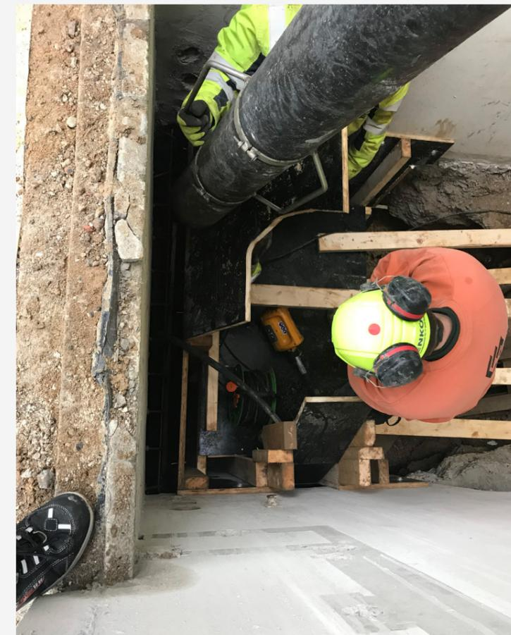
The process of fitting a new elevator shaft in the building to make it more accessible.
