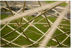
In 2016, to mark the Festival of Making in Sheffield, UK, a lightweight gridshell was designed and built. In collaboration with Swiss and Dutch engineers and architects based then at ETH Zurich, the 10m x 10m doublecurved structure was constructed by students
